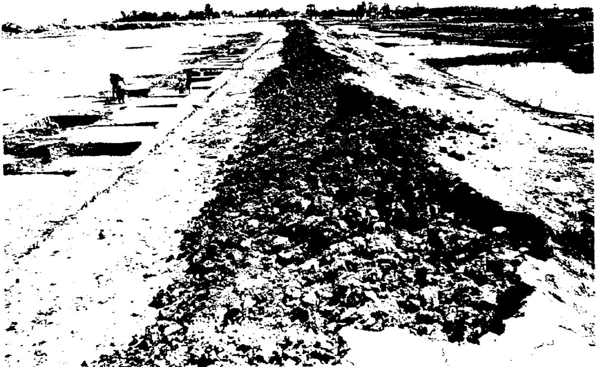
*Plate 3. Repair of a damaged sea-facing section of the earthen marginal embankment, Shibpur 'mouza' of southern Sagar, by replacing the eroded materials with chunks of clay dug from the intertidal mudflat.*
