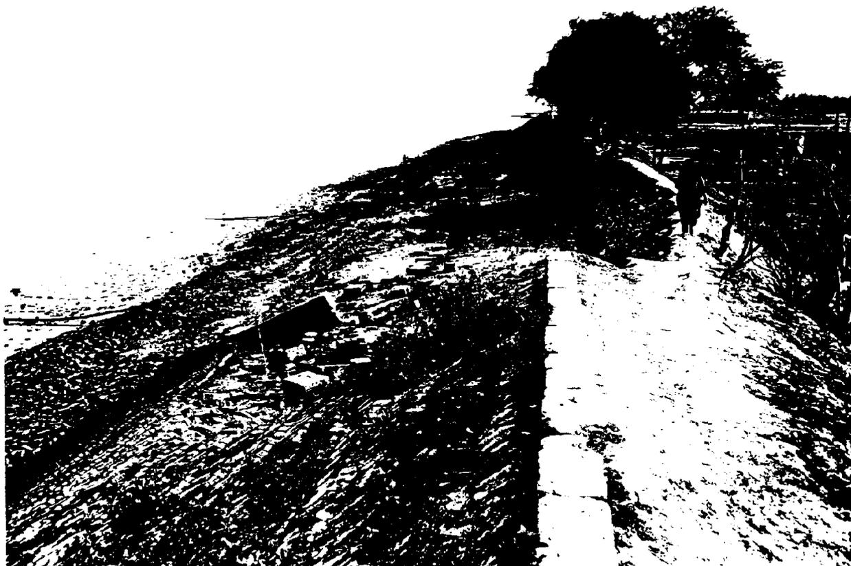
*Plate 4. Brick paving over earthen embankments in exposed sections of the coast, e.g. in the Kachuberiya ‘mouza’ of northern Sagar, can successfully prevent seasonal erosion in most cases but, once damaged, their repair may take a considerable time.*
